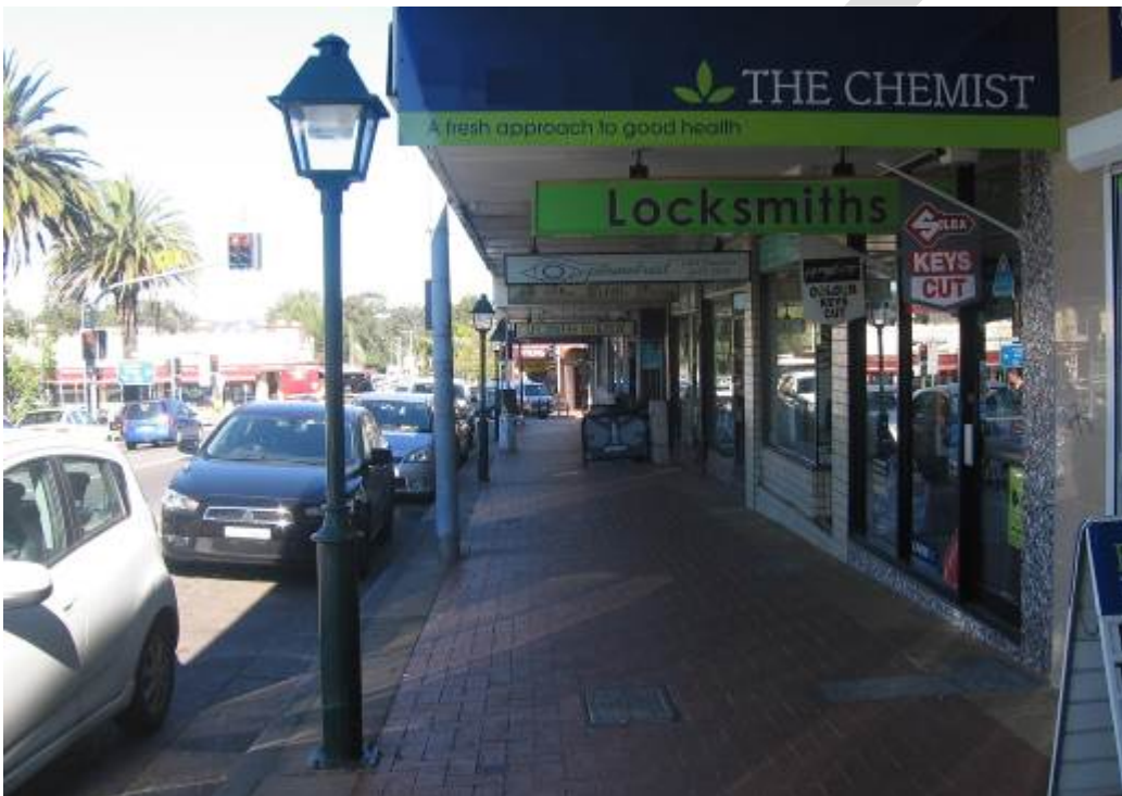
Figure 26 Example of buildings creating a consistent edge along the Pacific Highway
