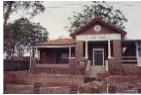
Former Court House
