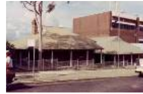
Police Station and Quarters
