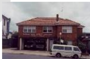
Brisbane Water Ambulance Station, Pacific Highway
