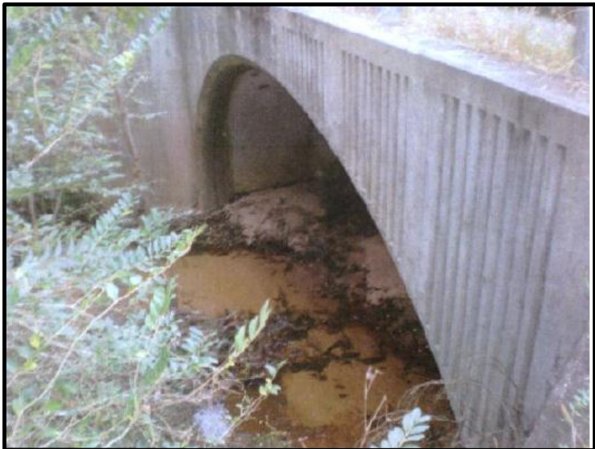
Plate 7 Arch culvert draining water beneath Ourimbah Creek Road
