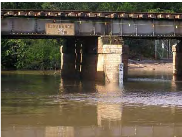
Turpentine Road underpass of Railway Line
