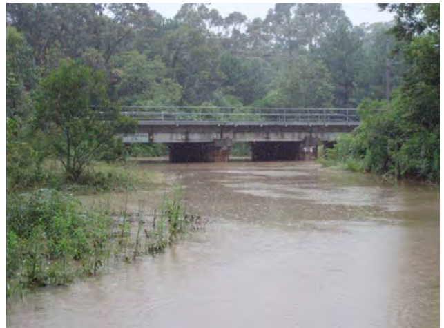
Turpentine Road underpass of Railway Line
