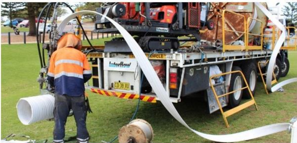
Photo line: 1 broken man hole and repaired and raised manhole from the reveal and seal program, 2 cracked and collapsed sewer pipes which have been fixed, 3 root intrusion, 4 pipe relining.
