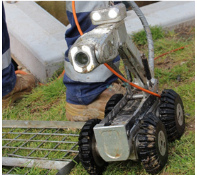
Photo 2: CCTV inspection camera
