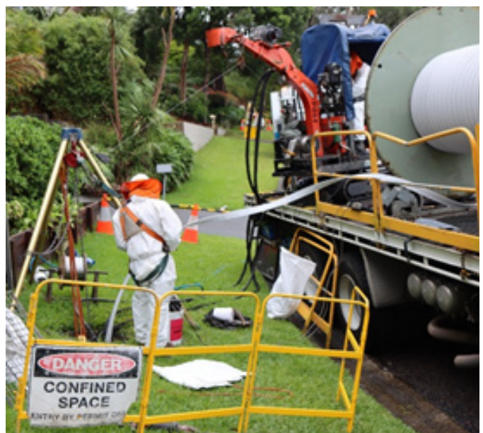
Photo 3: Pipe relining process
