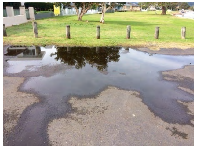
Davistown Progress Hall following heavy rain in March 2018
