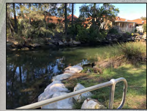
Existing Canals to be utilised for drainage connections
