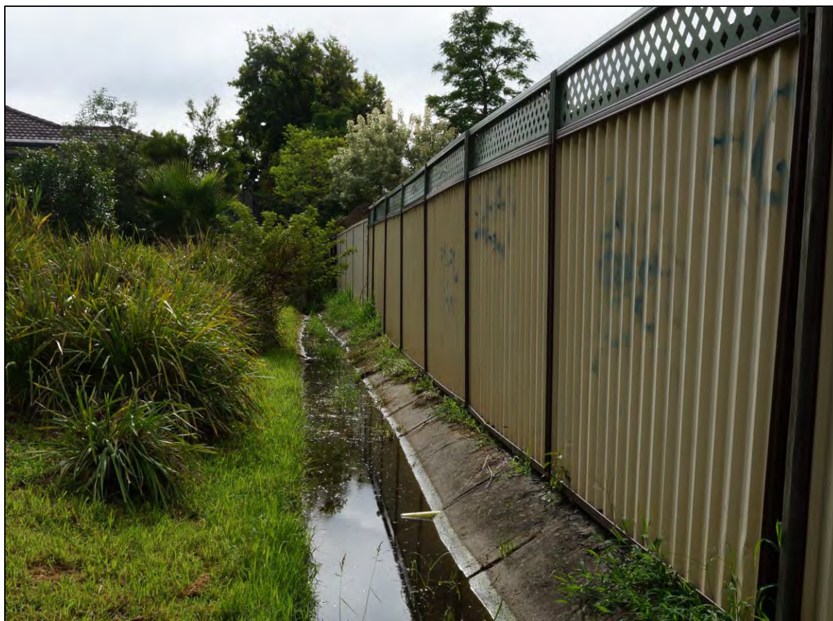
Plate 30 Allambee Crescent Drainage Channel
