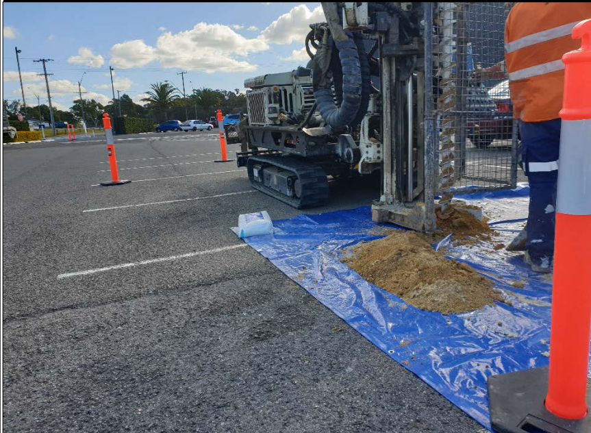
PHOTO 19: 49-65 WENTWORTH AVE – SHOWING INSTALLATION OF MW02 AT BH002, FACING NORTH, PHOTO TAKEN 12/08/2019
