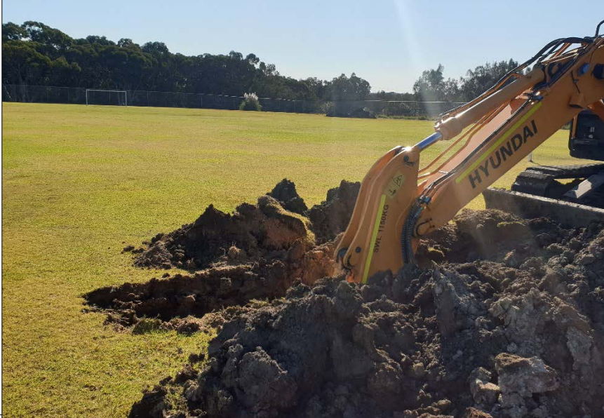
PHOTO 13: FILL FROM TP008 IN THE SOUTHERN PORTION OF SPORTS FIELD, WHICH INCLUDED A LARGE VOLUME OF DEMO WASTE AND ENGINE PARTS, 13/08/19
