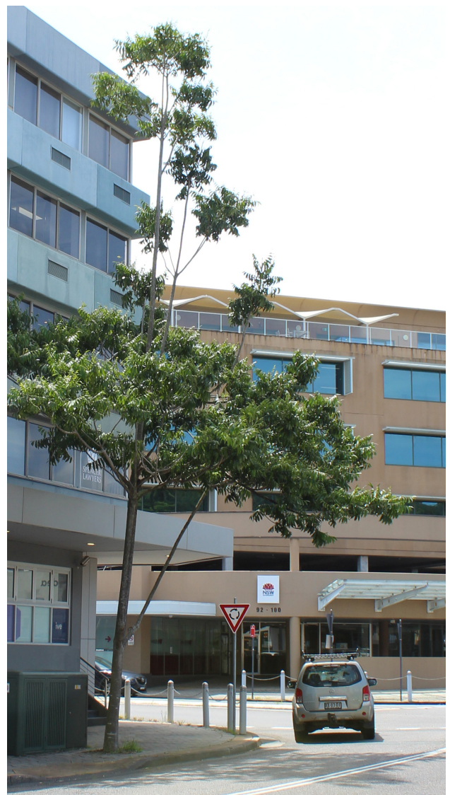
Inadequate space above ground
